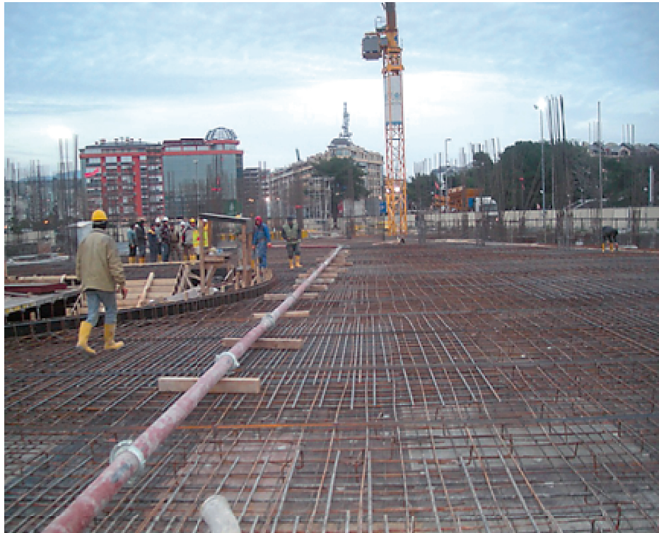
Figure 1: Preparation for concreting of reinforced concrete slab, pipes of stationary pump
